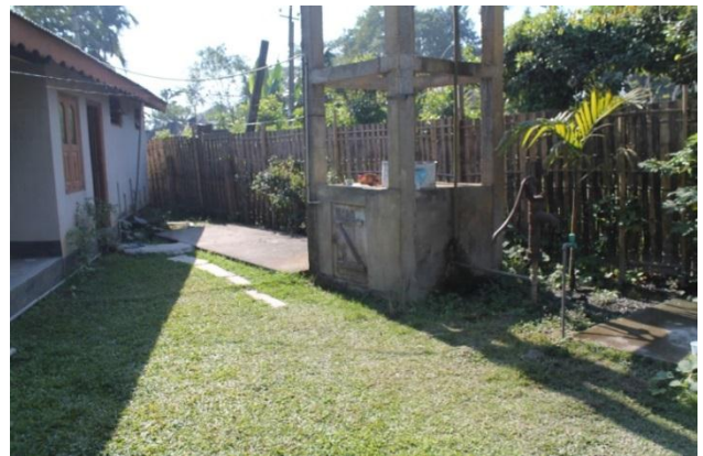
Figure 1-8: Example of water contamination by septic tank and water pump placed side by side.
