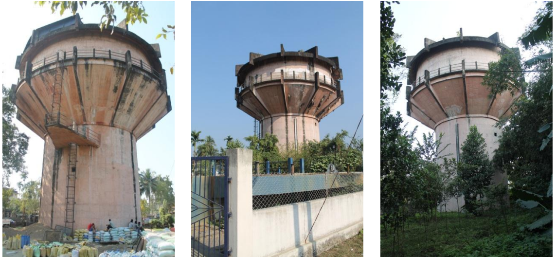
Figure 1-7: Elevated service reservoirs in Zones 1, 2 and 3.
