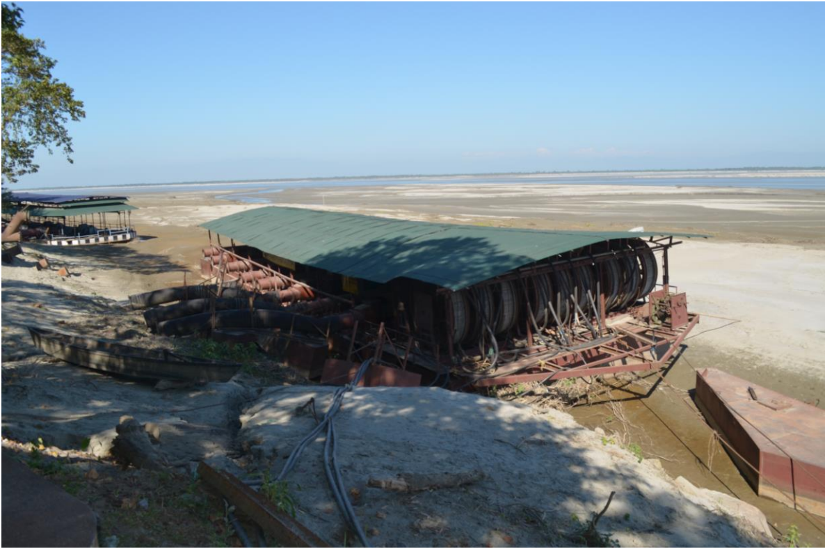
Figure 8-6 Barge mounted pumps at the Brahmaputra River (photo: LBG-DHI Nov 2013)
